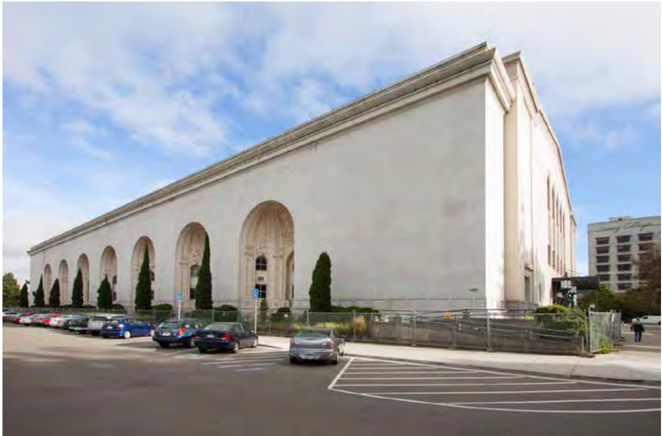
CA Alameda County Oakland Auditorium 0013 - North and West Exterior, 2017
