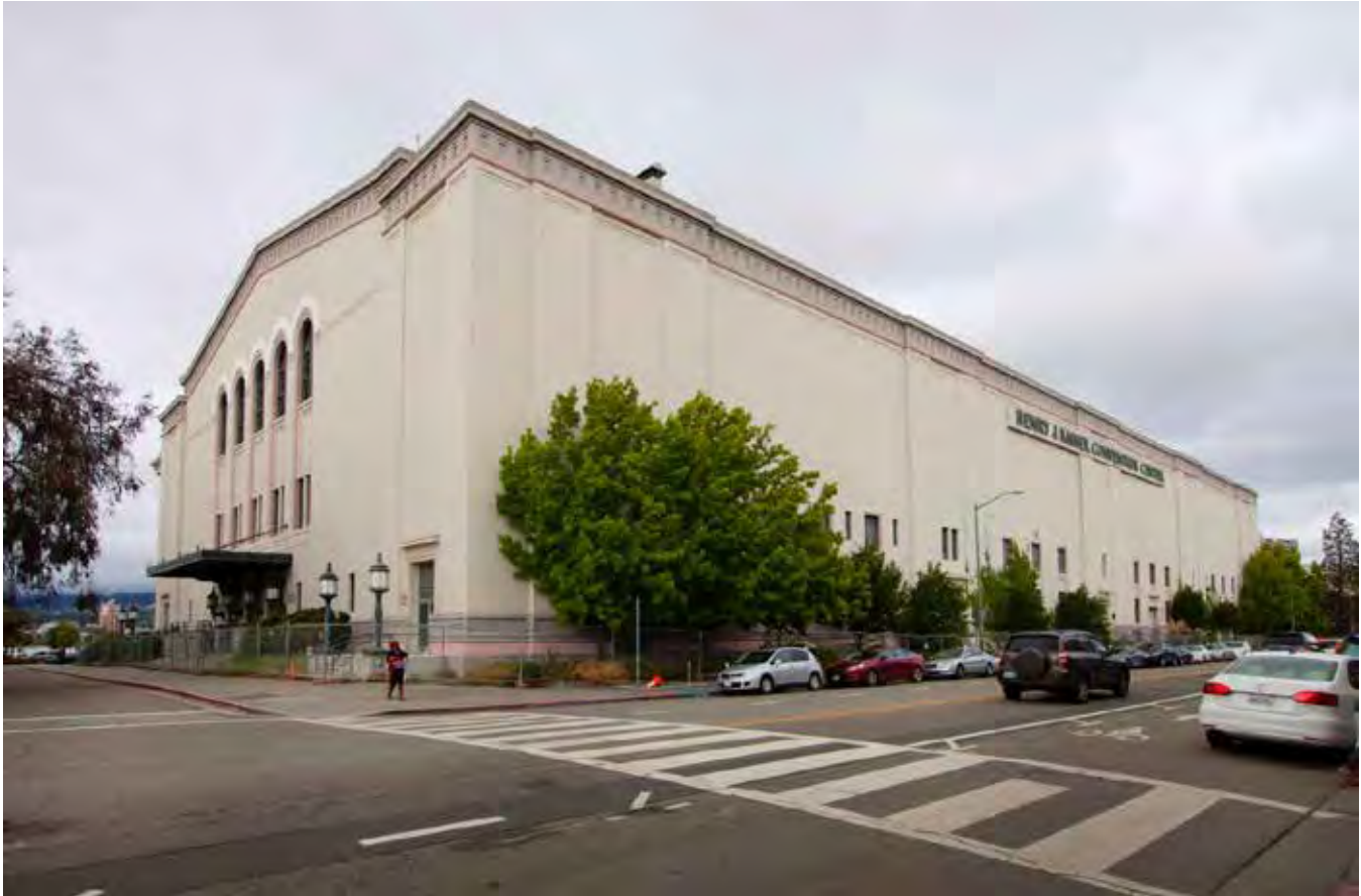
CA Alameda County Oakland Auditorium 0014 - West and South Exterior, 2017
